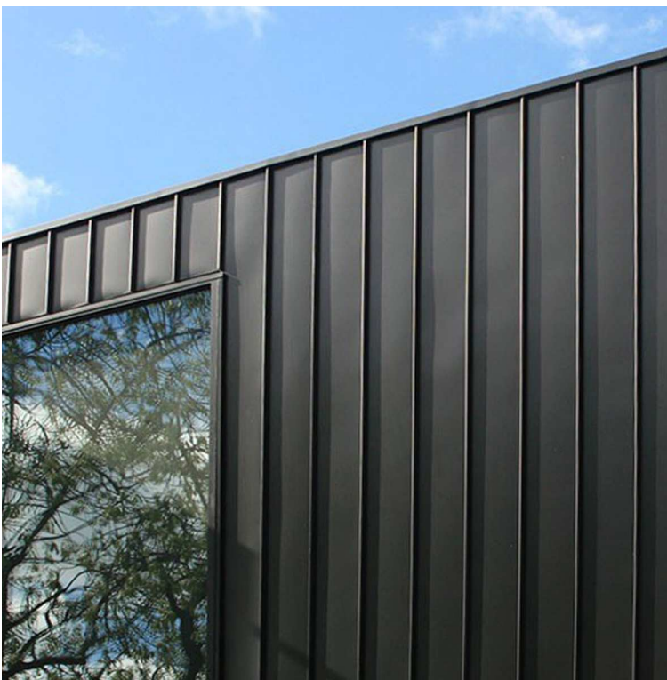
PROFILED METAL WALL SHEETING
