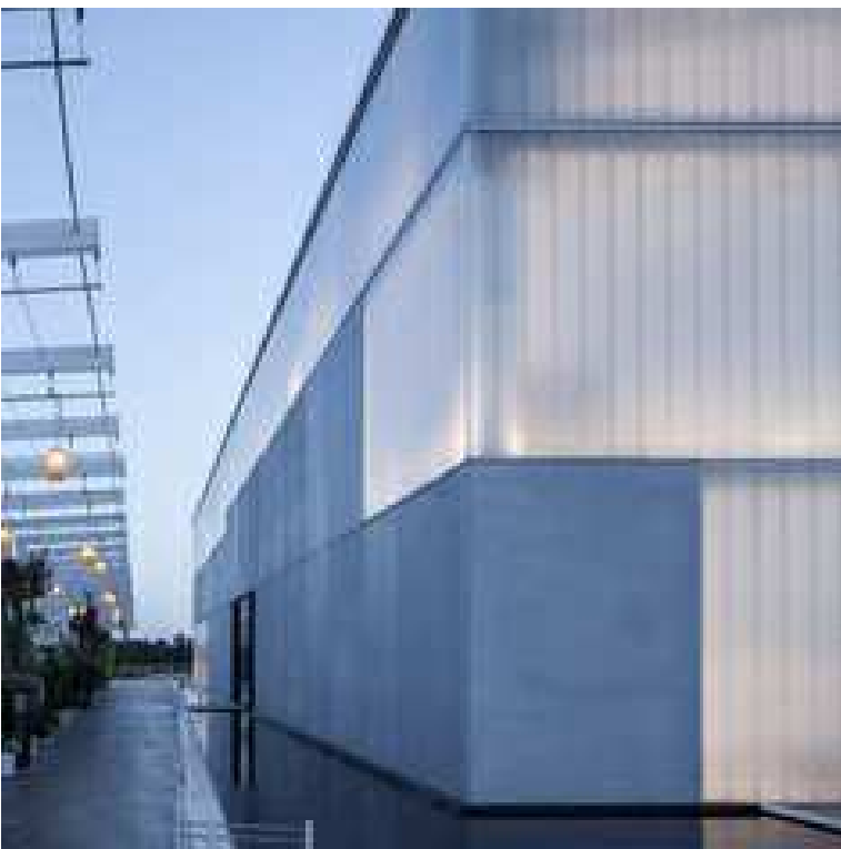
TRANSLUCENT PROFILED WALL SHEETING
